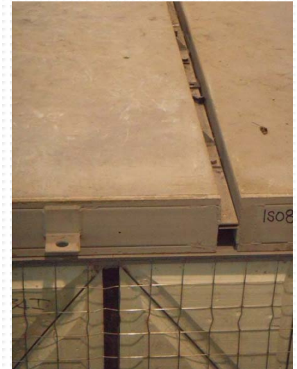
Cross section showing the upper & lower (floor/ceiling) U channel separated by a rigid rubber strip for sound & water proofing. Moreover, it will be a great spare access for any future MEP alterations. This gap will be finally filled with plaster for fire resistance.
