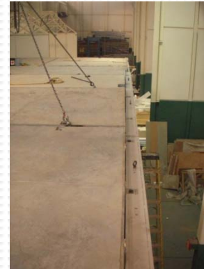
Good fit for the last floor panel of this section
