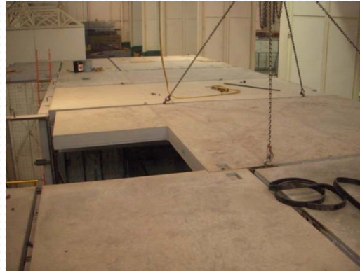
Good fit for the last floor panel of this section
