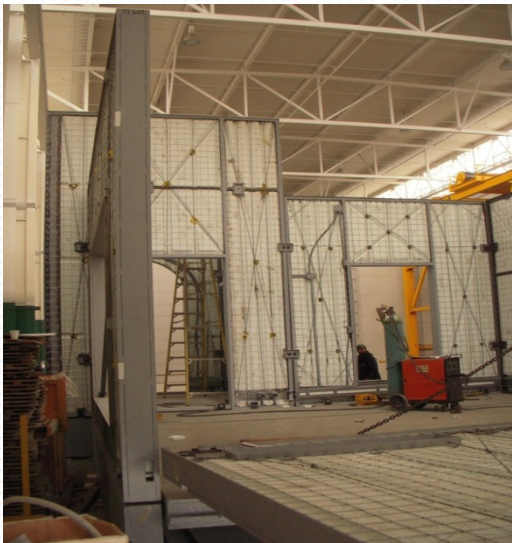
DRY RUN ASSEMBLY OF THE THIRD SECTION OF THE SHOW HOME, SHOWING VARIOUS ON-GOING INTERESTED DELEGATIONS
