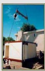
ERECTION OF LARGE KITCHEN 3-D MODULE USING 2 MOBILE CRANES.
