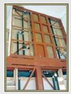
INTEGRATED WATER/DRAINAGE PIPES INTEGRATED IN THE PANELS ACCESSIBLE FOR MAINTENANCE (EXPOSED FOR VIEWING).
